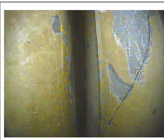
Figure 6. Post-test videoscope inspection (side view) at bundle elevation 790 mm.
