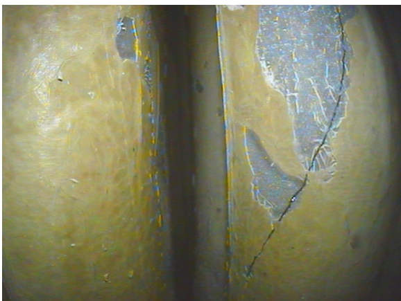
Fig. 7. Post-test videoscope inspection (side view) at bundle elevation 790 mm: spalling of nitride containing oxide scales.
