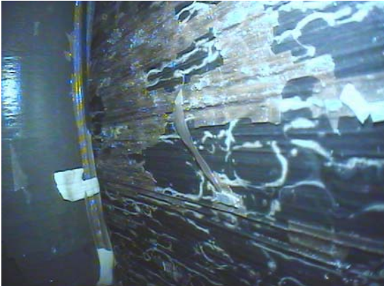
Fig. 12. Videoscope photograph with a side-view lens at elevation of 0.70 m: intensive oxide scale spalling on the coarse shroud surface.
