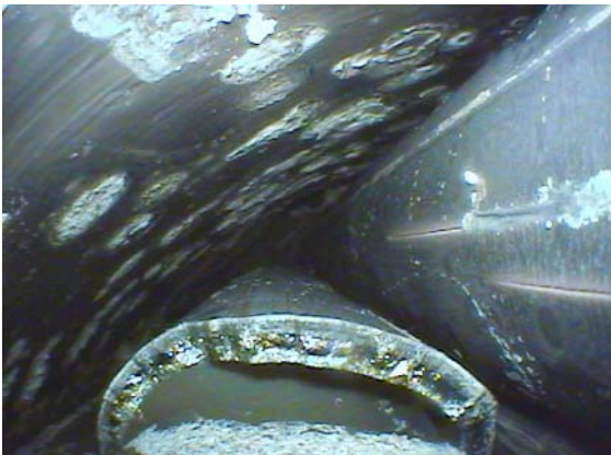
Fig. 13. Videoscope photograph at elevation of 0.90 m: circumferential and longitudinal cracks at the cladding; nodular breakaway corrosion at the shroud.
