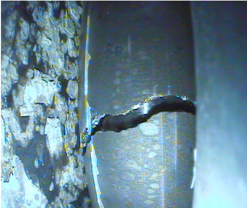
cross crack at 600 mm (rod D)
