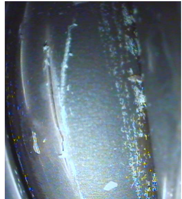
longitudinal crack at 650 mm (rod F)
