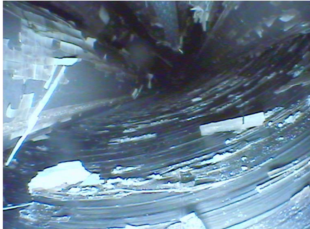
camera in position of corner rod D at 650 mm: spalled oxide scales at shroud and cladding
