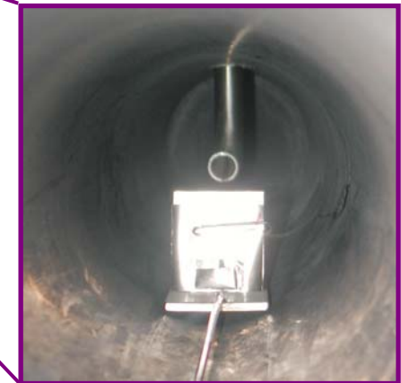
Ni-plate with pocket installed inside off-gas pipe under sampling tube
