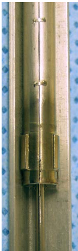
TC fastening at outer surface of cladding
