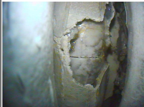
600 mm: damaging of cladding due to influence of melt
