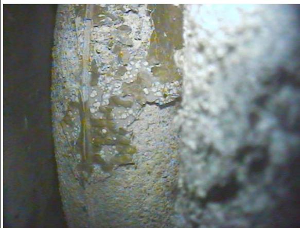
775 mm: spalling of outer oxide scales
