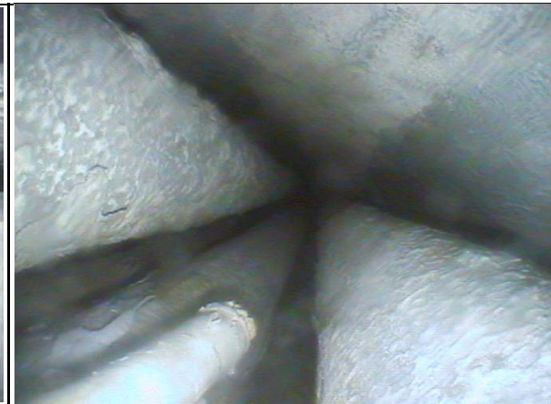
650 mm: absence of upper spalled oxide scales
