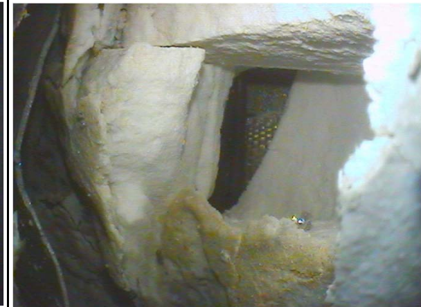
550 mm: ZrO 2 insulation damage under failed shroud
